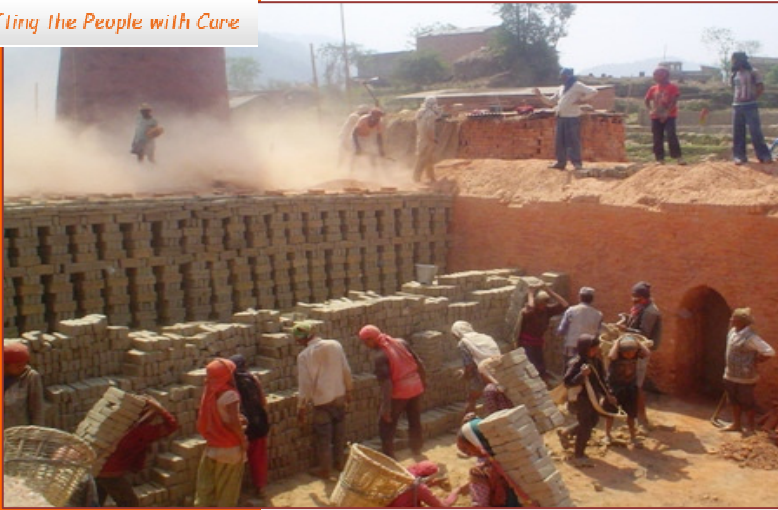
Worker carrying bricks and arranging bricks for baking
